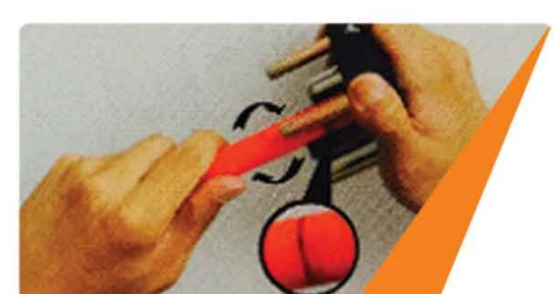
3.Make sure the accessories of the fitting is complete, and insert the tube into the fitting until it reaches the block area. Be sure the marks on the pipes are even with the ends of the fitting.
